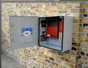
Rack Enclosure mounted on a wall
